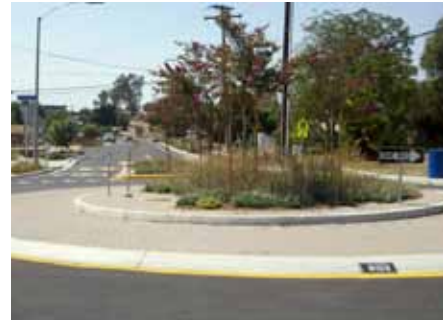
Rock Springs Roundabout, before (top) and after (bottom).
